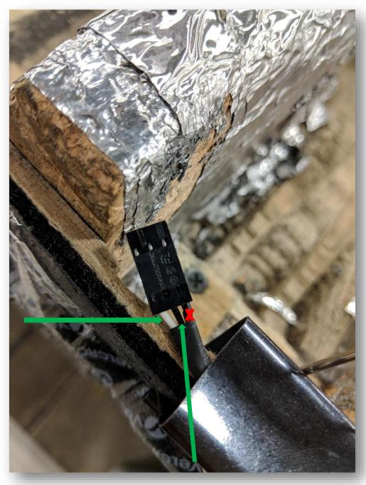
Locate Black and White Wires On Back Side of TSB Connector (Do not test shielded wire)
